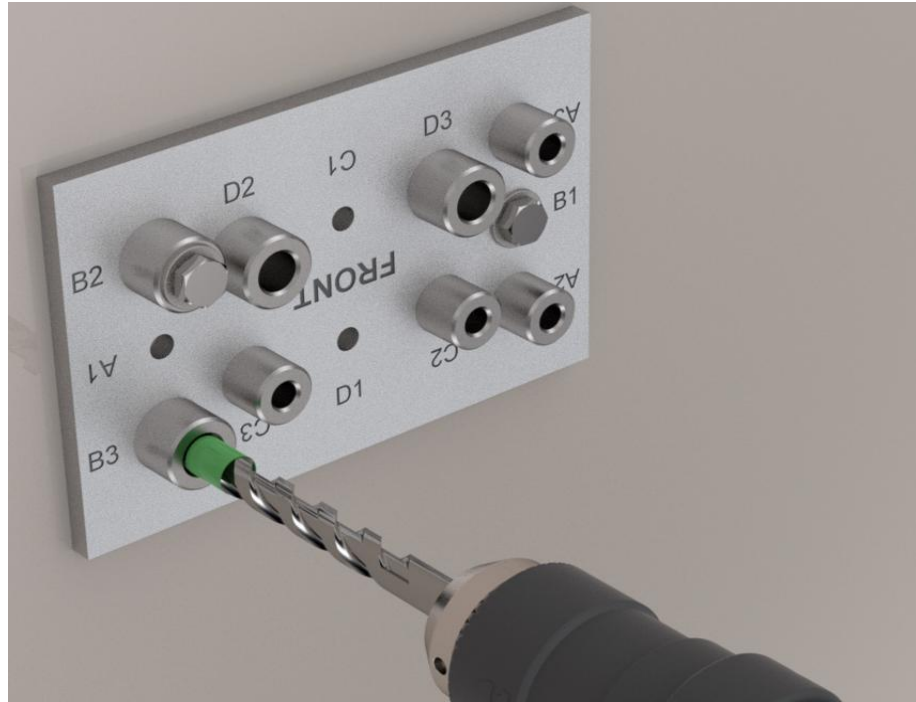
Figure 37: Drilling Third Hole Through Bushing B3 for Drop-In Anchor
