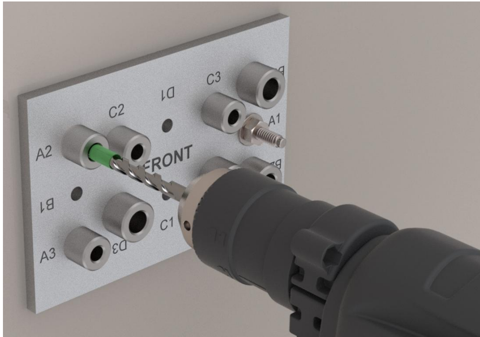
Figure 23: Drilling Second Hole Through Bushing A2 for Wedge Anchor
