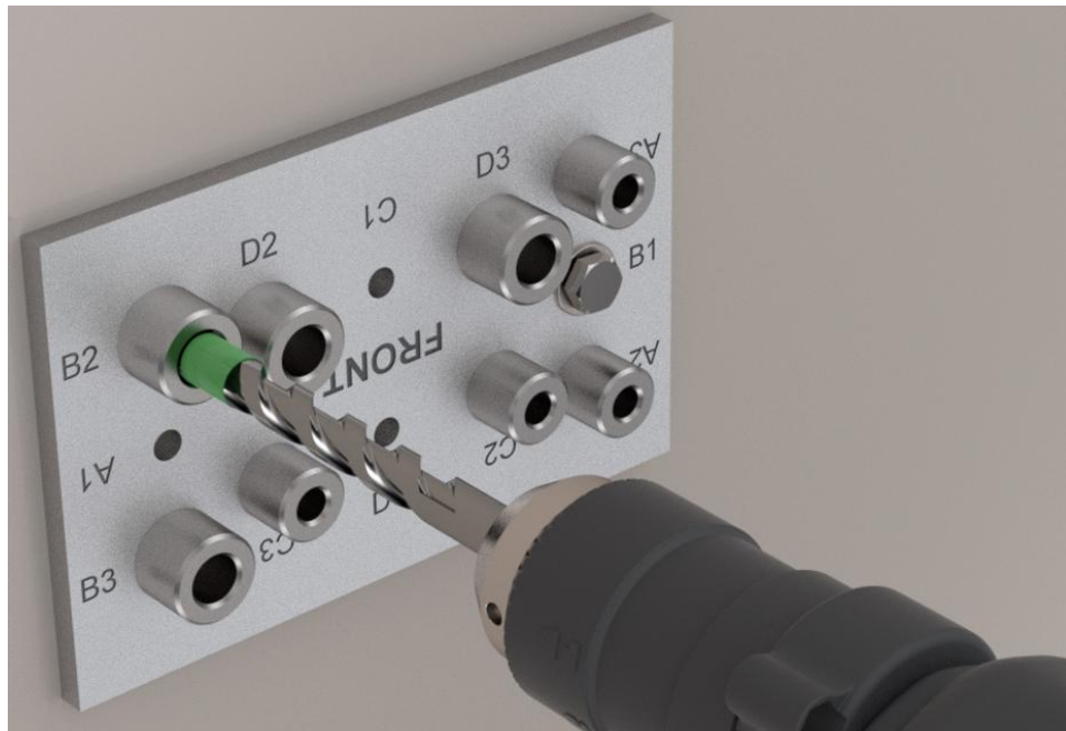
Figure 35: Drilling Second Hole Through Bushing B2 for Drop-In Anchor
