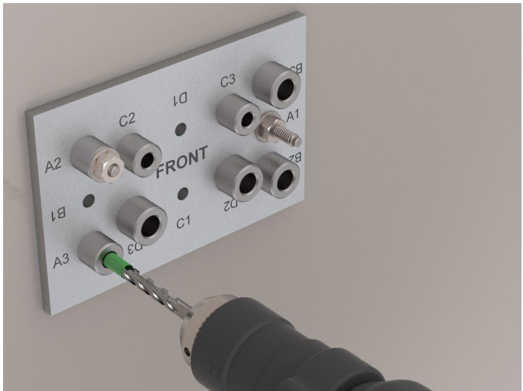
Figure 25: Drilling Third Hole Through Bushing A3 for Wedge Anchor
