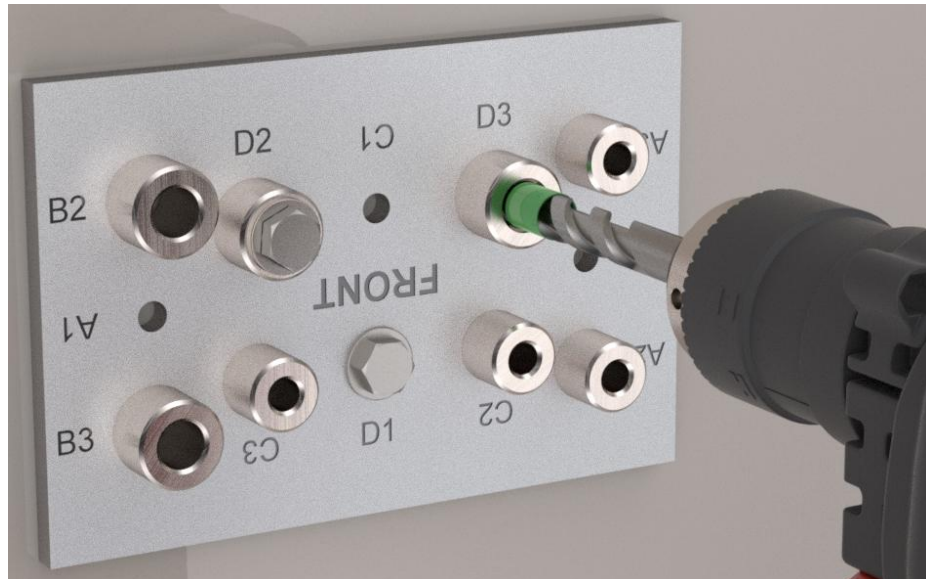
Figure 59: Drilling Third Hole Through Bushing D3 for Drop-In Anchor
