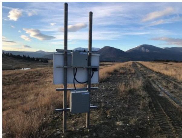
Figure 10: Example of Gateway Control Box Configuration Field Installation
