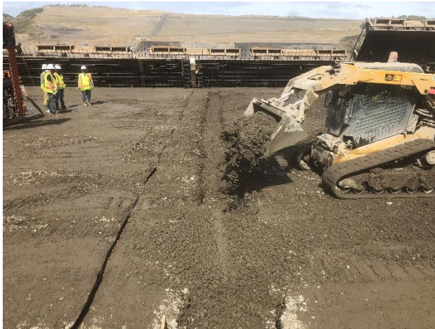
Figure 6: Applying the Embedment Material
