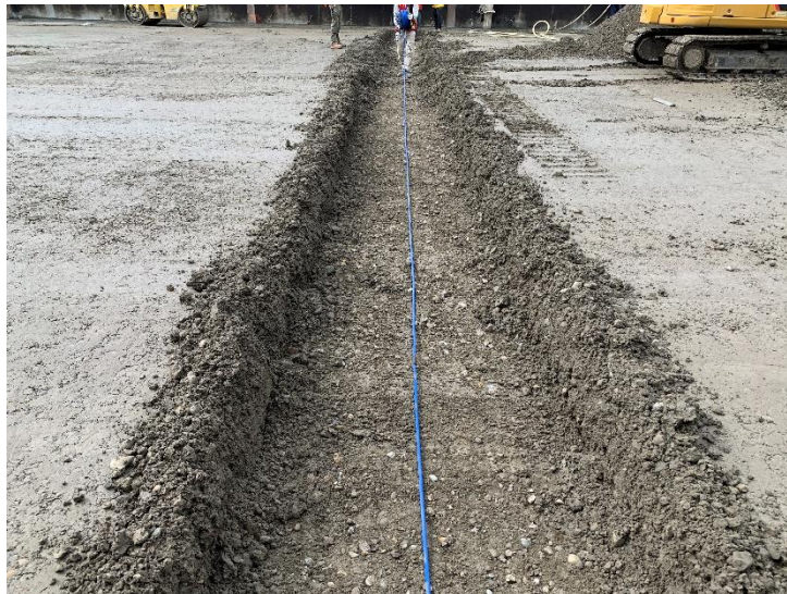
Figure 4: Laying the Thermistor String for Installation by Embedment
