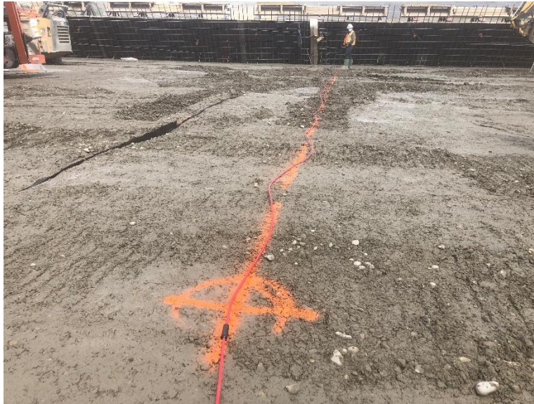
Figure 5: Marking the Positions of the Thermistor Sensors
