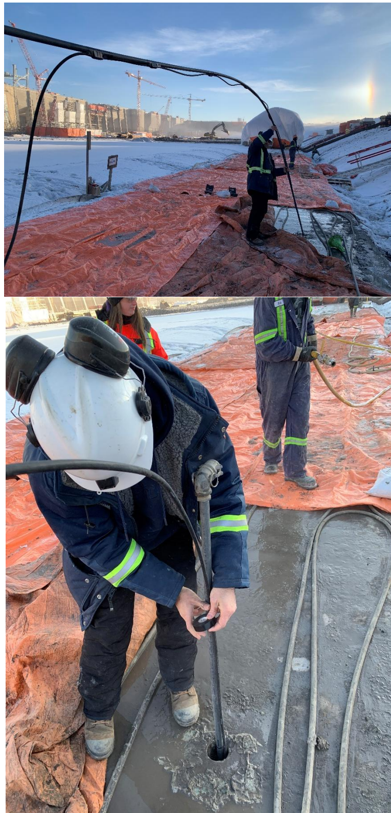
Figure 3: Lowering Thermistor String Assembly Attached to Sacrificial Tremie Pipe Down the Borehole
