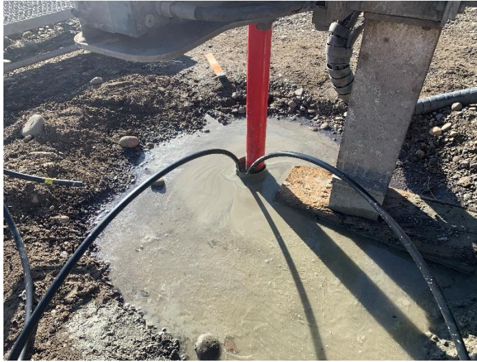
Figure 12: Pumping Grout through the Grout Pipe to Set the Casing Assembly in Place
