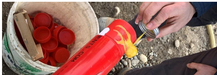
Figure 5: ABS 771 Cement Application Around the Male End of the Casing
