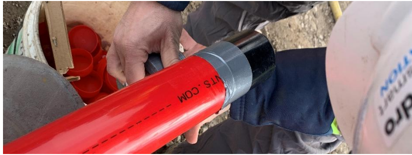
Figure 6: Attaching and Securing the Bottom Cap to the Casing
