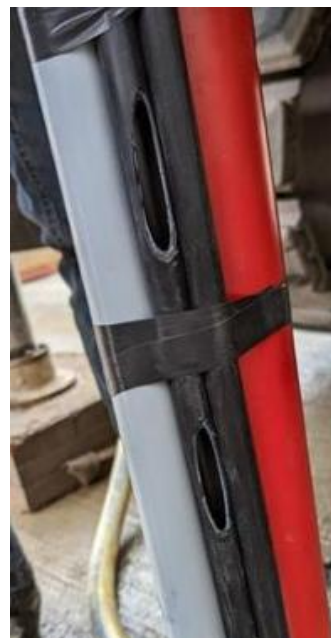
Figure 7: Attaching a Grout Tube to the Casing
