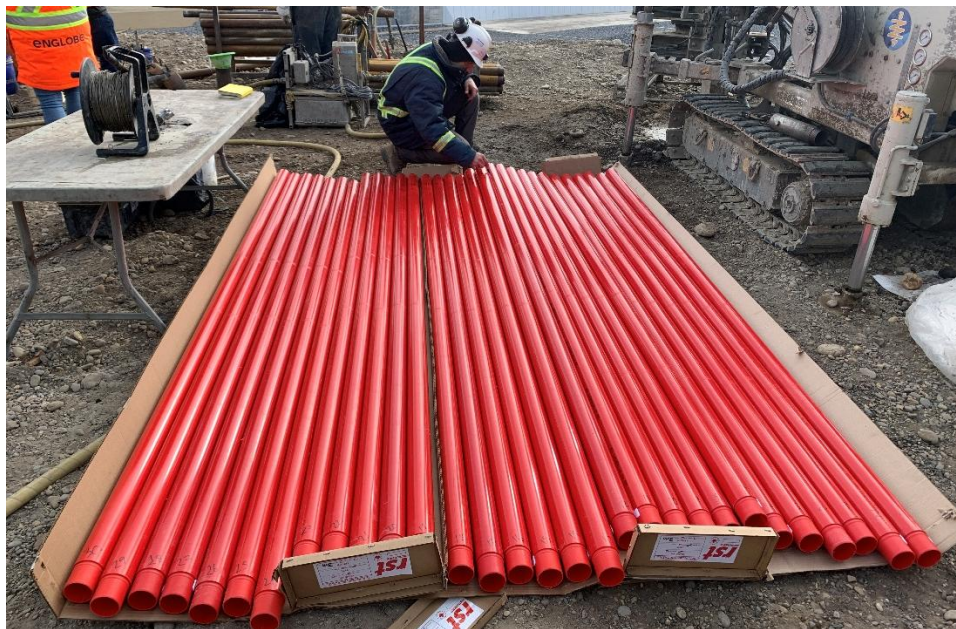
Figure 3: Visual Inspection and Marking of Casings
