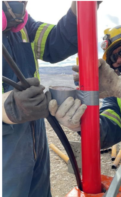
Figure 7: Attaching a Grout Tube to the Casing
