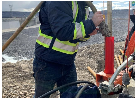
Figure 11: Filling the Casing with Clean Water to Neutralize Buoyancy
