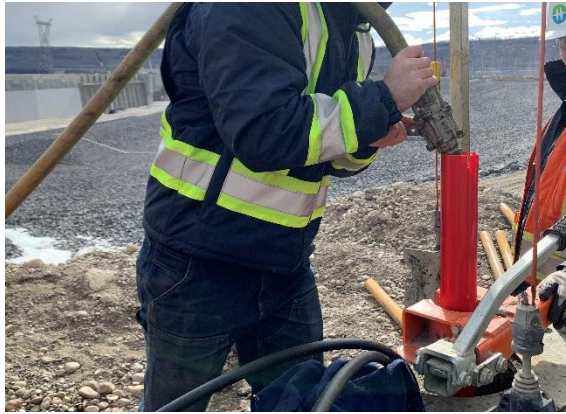
Figure 9: Filling the Casing with Clean Water to Neutralize Buoyancy
