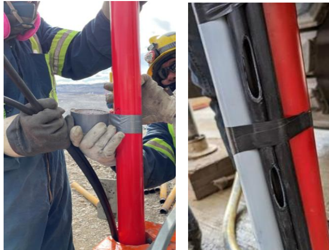
Figure 6: Attaching a Grout Tube to the Casing
