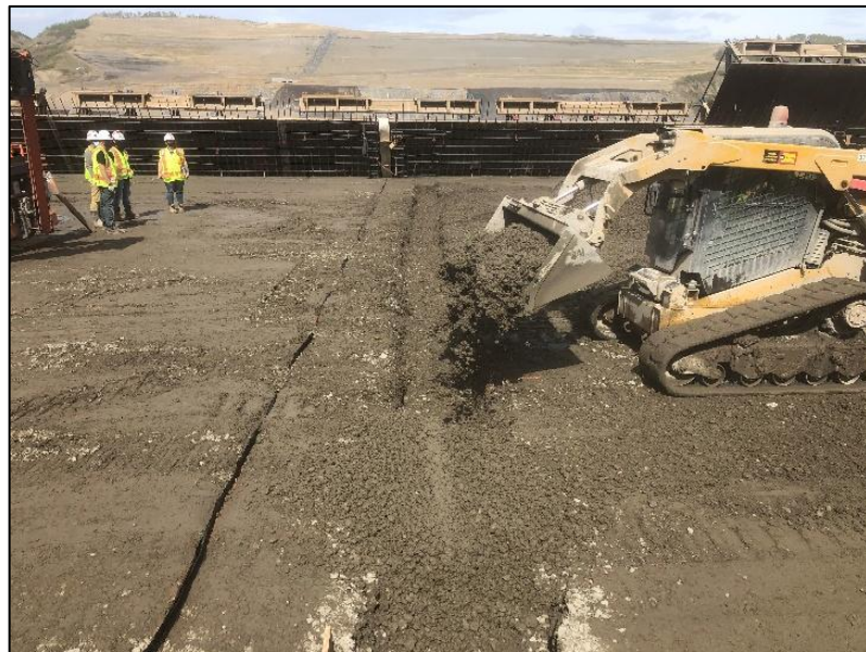
Figure 6: Applying the Embedment Material
