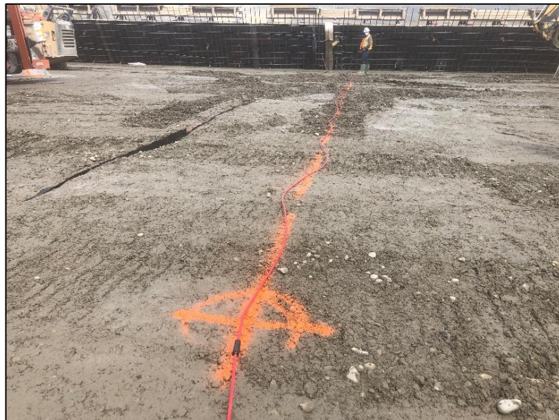
Figure 5: Marking the Positions of the Thermistor Sensors
