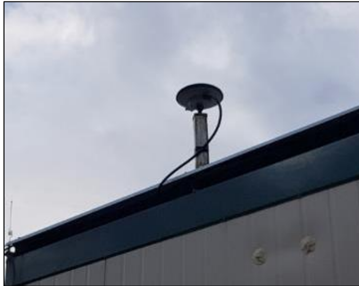
Figure 10: GNSS Antenna Example Installation
