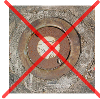
FIGURE 1-1 DATALOGGERS SHOULD NOT BE INSTALLED IN WELL COVERS
