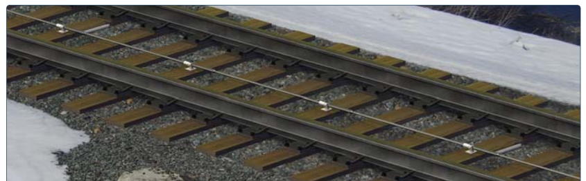
Above: Increasing close-up images of a bussed section along the Track Monitoring System. Below: A portion of railroad track showing an installed Track Monitoring System.
